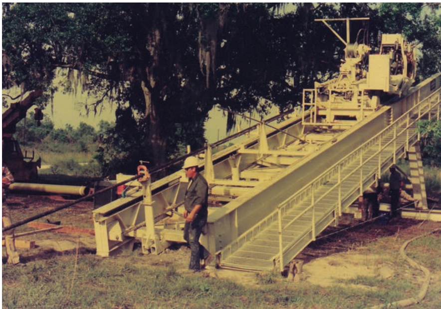
↑ Cherrington's first HDD rig was built for a river crossing, shown here working on a series of river crossing projects in the 1970s.
