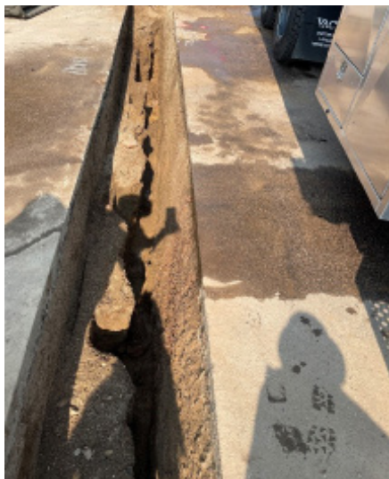
Slot trenching to find unmarked utilities for future.
