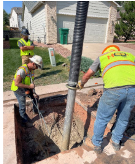
HCD locating a gas main for Colorado Springs Utility could pressure test the line.
