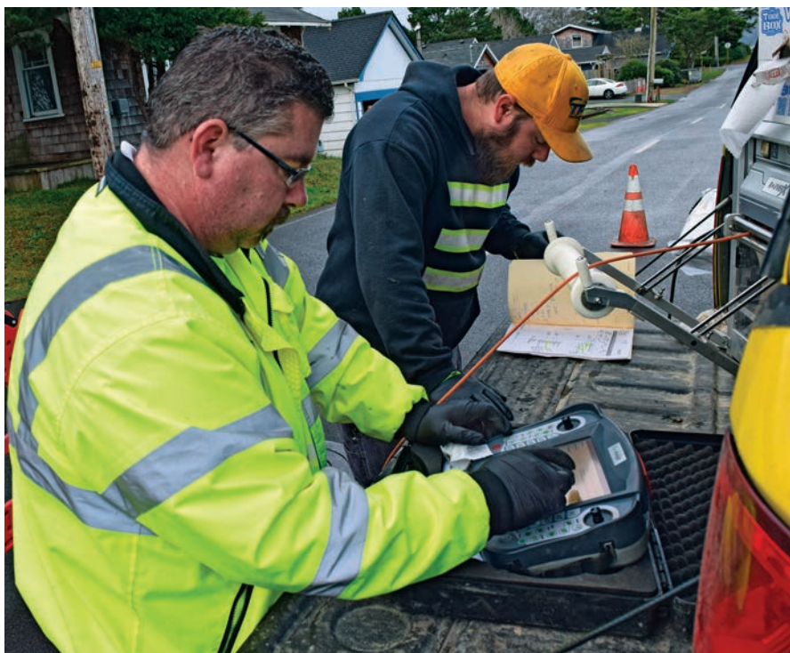
Trenchless Pipe Repairs captures video and enters defect codes into the ROVVER X's handheld touch screen controller. Once the lines are televised and the crew's observations are entered, a finished report can be generated.
