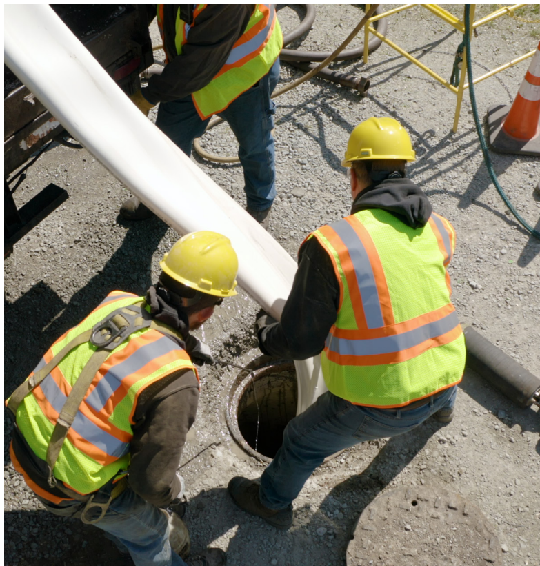
NovaForm is heated and conditioned at the job site using steam and then pulled from reels by high-powered winch into an existing sewer/stormwater pipe that remains buried.
