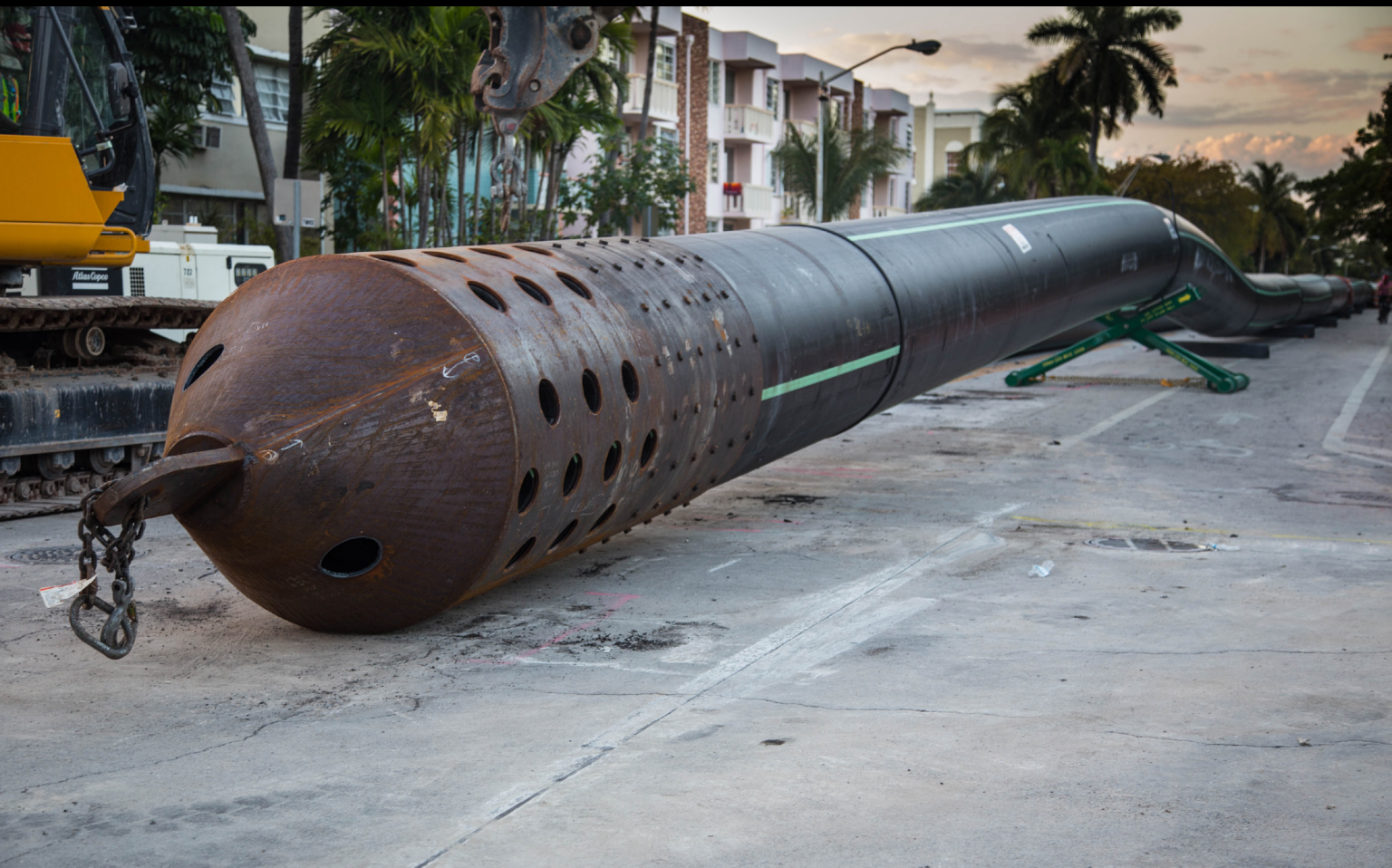
Miami-Dade Sewer Force Main rehabilitated with more than 4,000 feet of 54" HDPE pipe, installed using Horizontal Directional Drilling.
