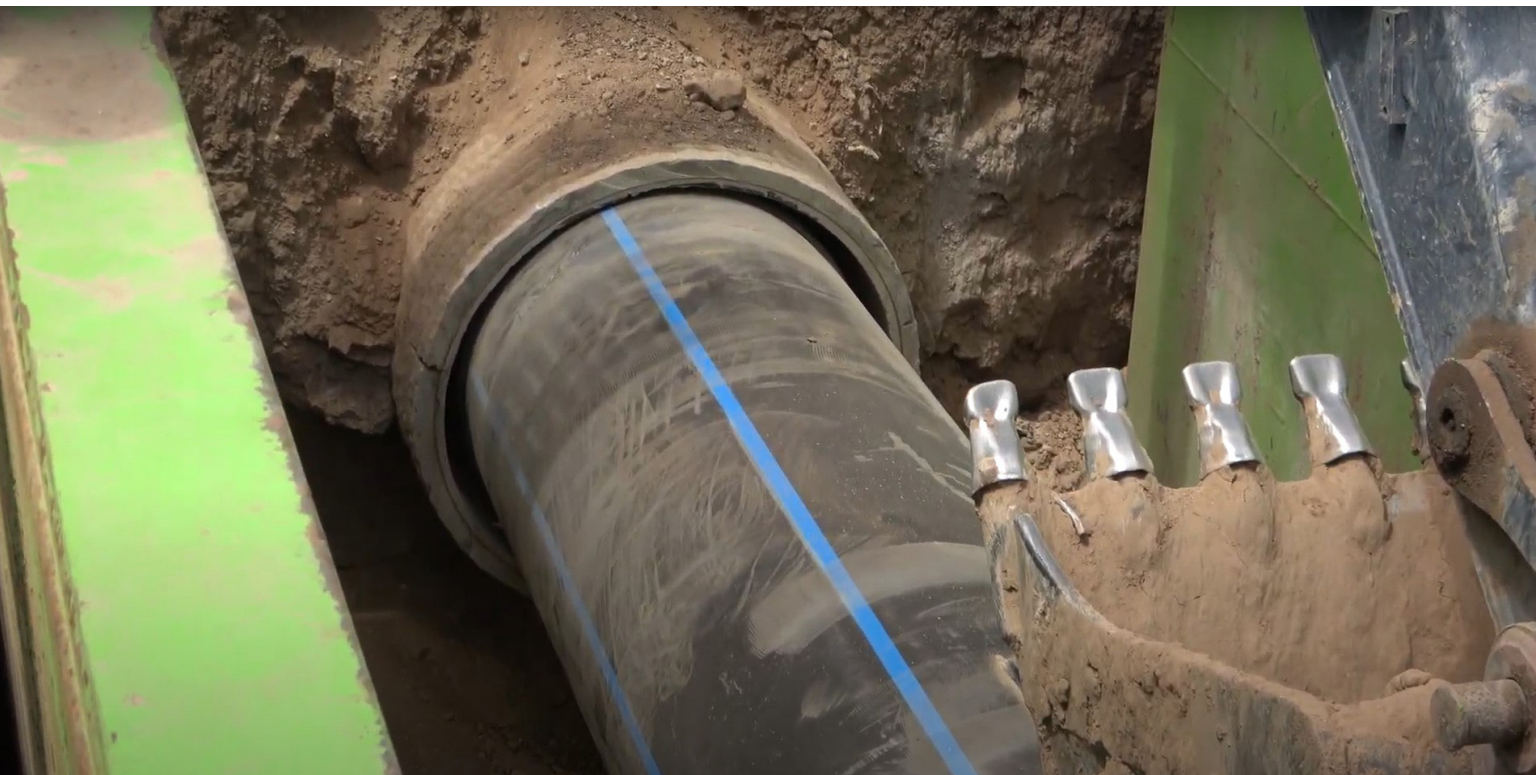
Tucson Water Sahuarita Supply Line rehabilitated using 32" HDPE DR 21 pipe, installed via sliplining trenchless method.
