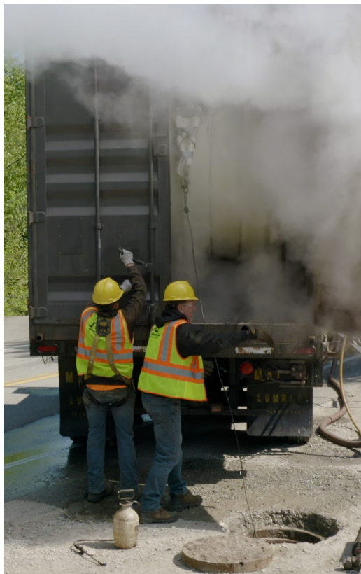
NovaForm is heated and conditioned at the job site using steam and then pulled from reels by high-powered winch into an existing sewer/stormwater pipe that remains buried.
