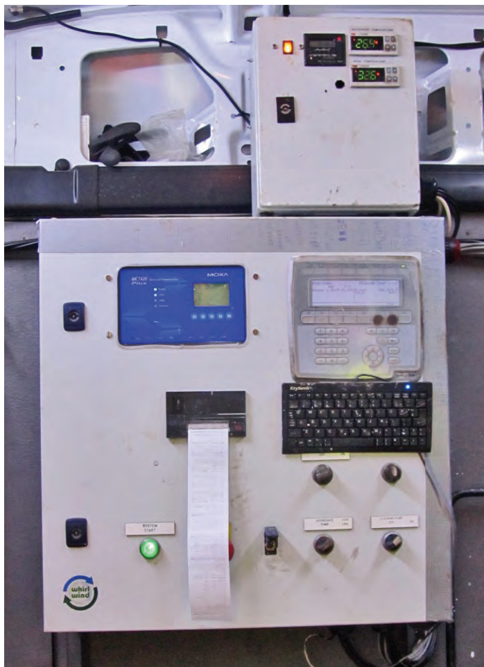
The Serline system is controlled by computer and sensors throughout the system relay temperature, air flow and other information to field crews to give real time data reporting.
