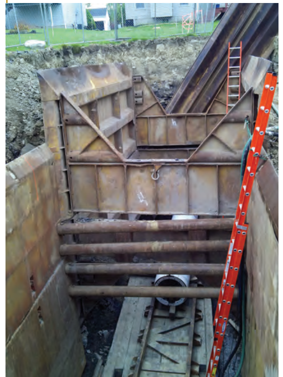
THE ROBBINS SBU-RC WAS LAUNCHED FROM A 23-FT DEEP BORE PIT IN THE BACKYARD OF A HOUSE PURCHASED BY THE PROJECT
