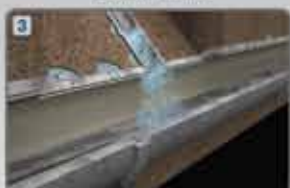
Continues to leak in annular space
