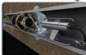
Leaking joint in mainline sewer
