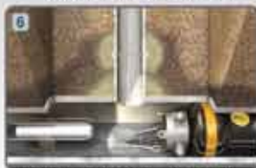
Grout collar stops infiltration
