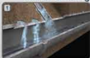
Leaking lateral
