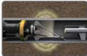
Grout collar stops infiltration
