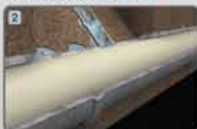
Liner installed
