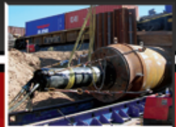
PIPE RAMMING/HDD ASSIST
