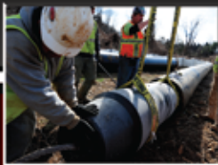
PNEUMATIC PIPE BURSTING
