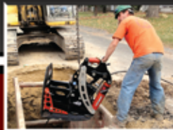
LATERAL PIPE BURSTING
