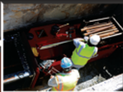
STATIC PIPE BURSTING
