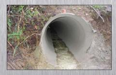
gated metal pipe invert repair is for structural refurbishment of damaged inverts common in culverts. PL-12,000 is placed by spinning the mortar to conform to the radius of the invert without affecting the flow characteristics of the existing culvert.
