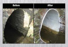
mance benefits of TPU including abrasion and chemical resistance, and low temperature flexibility. Traditional and less expensive systems use styrene as a crosslinker for curing resins, but the drawback is the strong odor and contaminated water that requires special disposal, resulting in additional costs. Listening to the installers, it became apparent that finding a solution
