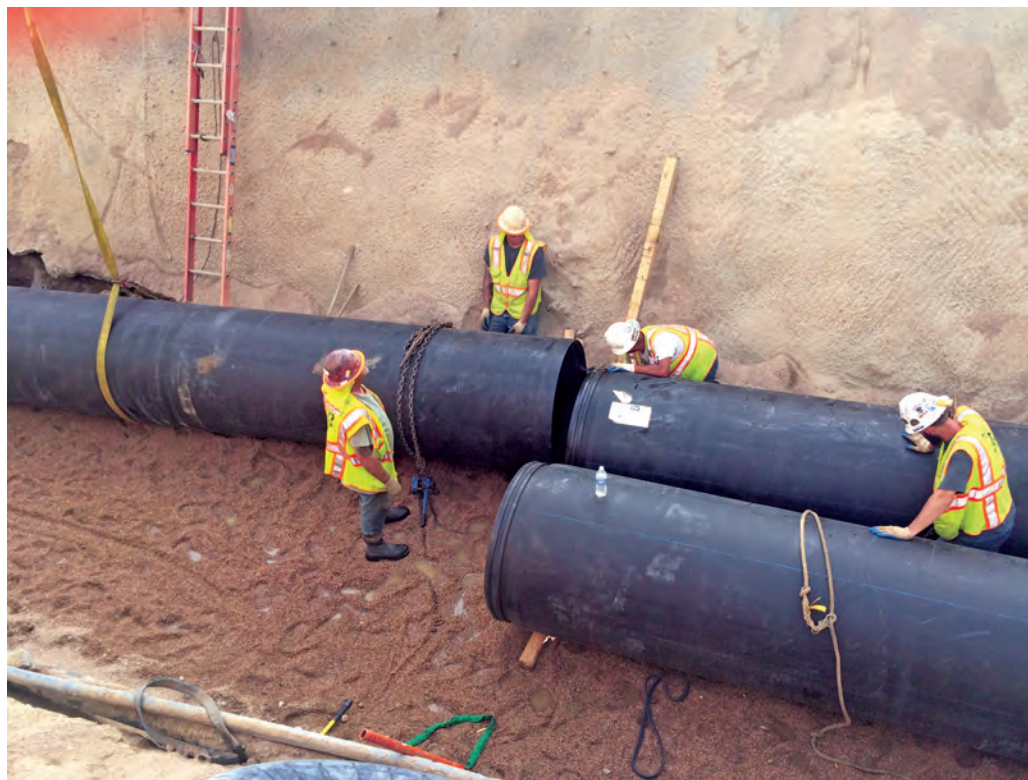
THE PIPES WERE CONNECTED TO AN EXISTING CONCRETE COLLECTION VAULT THEN RAN 120 FT WITH THE LAST 40 FT UNDER AN ACCESS ROAD BEFORE DISCHARGING TO AN OPEN STORMWATER DITCH.
