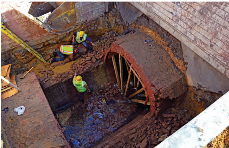
INSPECTION OF THIS SEGMENT OF THE DRAIN IDENTIFIED CRACKS AND DEFORMATIONS TO THE CROSS SECTION ABOVE THE SPRING LINE, AS WELL AS MISSING BRICK AND MORTAR IN THE CROWN AND INVERT ALLOWING SOIL TO INFILTRATE INTO THE DRAIN.
