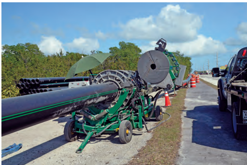
18-in. HDPE pipe was butt fused with McElroy's MegaMc 1236 and staged along U.S. 1.
