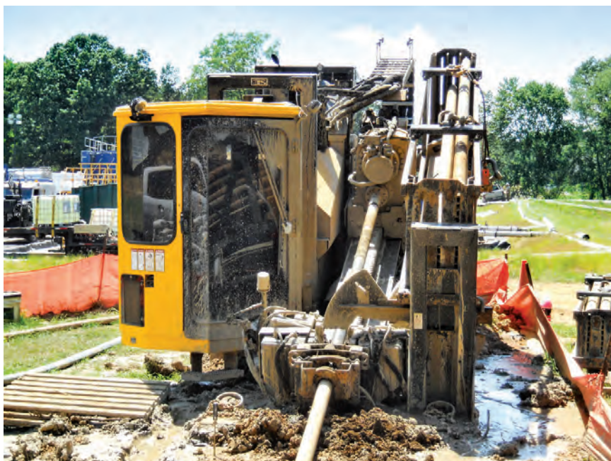
The drill plan specified a continuous bore of 1,170 ft that included a 100-ft underground river crossing — at a depth of 150 ft — approximately 480 ft into the route. Cline Trenching used a Vermeer D80x100 Series II drill.
